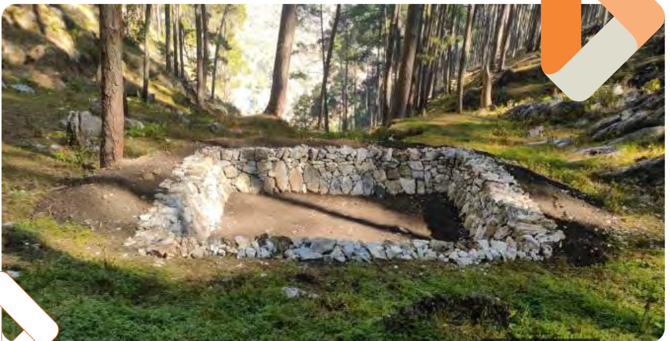
Percolation Pond 1 at Munakot
